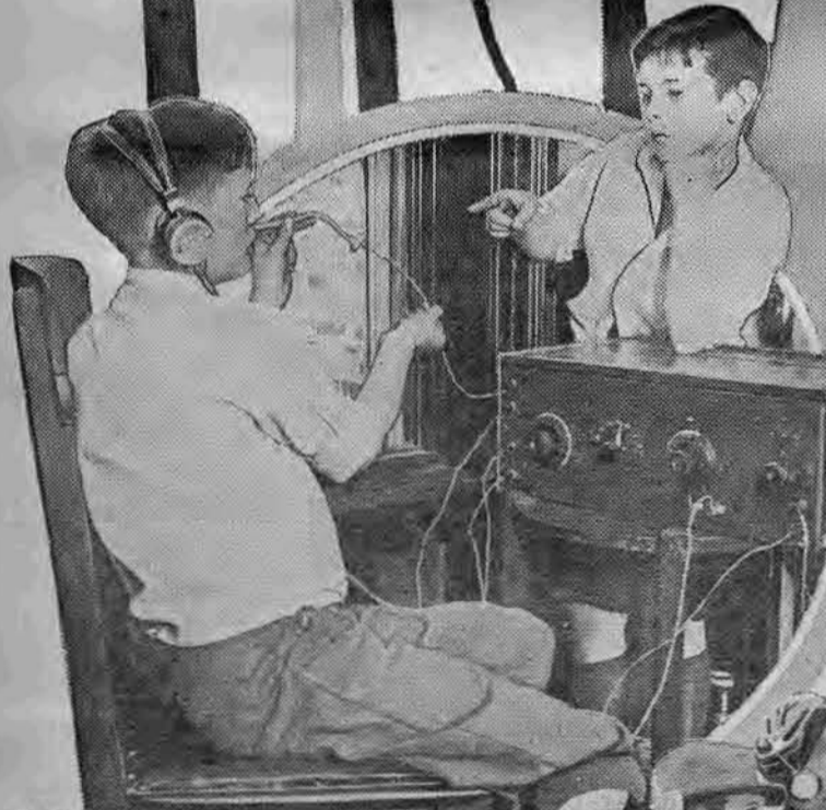
Receiving set made by Daniel Callahan. He had trouble with the landlord in putting up an aerial but now uses a wire clothesline instead. © K. & H.
